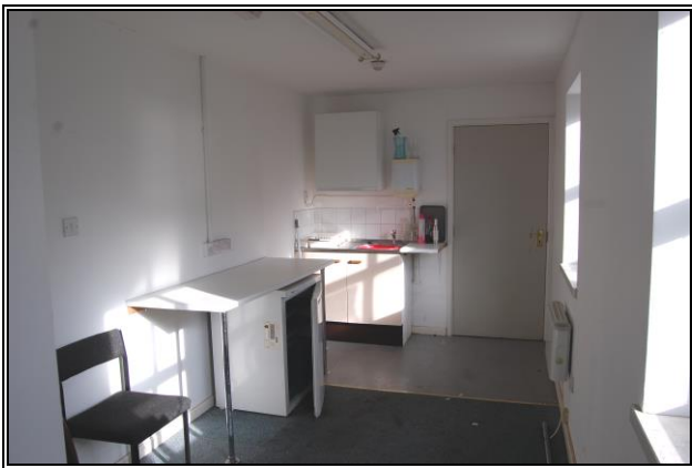
First Floor Staffroom / Kitchen
